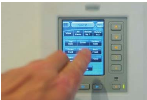
Above: an Audio Authority HD video distribution system is used for CCTV footage Below: CCTV can be controlled using this keypad Below, right: the long kitchen is a highlight
